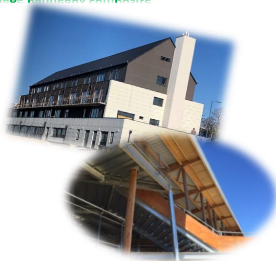
Restructuration du collège de Sancerre (18) Charpente -bois – ossature bois Bardage panneaux composite
